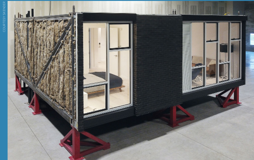
A “smart” apartment prototype on display in Skender’s Chicago factory. The steel-frame module uses the Z Modular/VectorBloc, a Lego-like steel connection system that “pins” the modules together.
